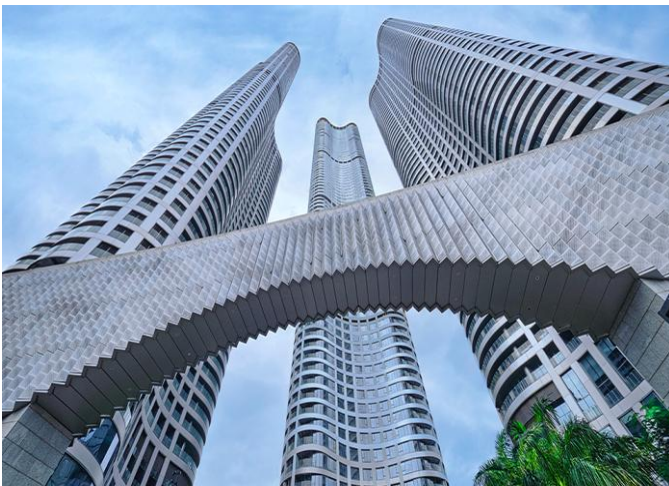
Exhibit 49: Lodha World Towers, Worli
